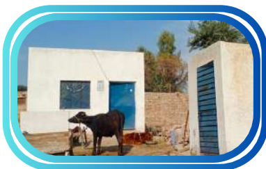
The shelter consists of a 14x14 ft living room, a Washroom and traditional kitchen (Choolha).
